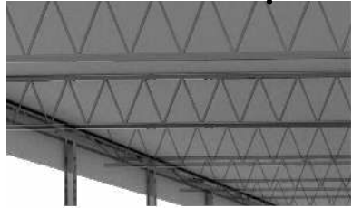
Flat surface truss system
